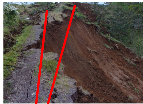
Fig. 6. "NE" direction cracks. San Miguel-Cariblanco-Cinchona area
