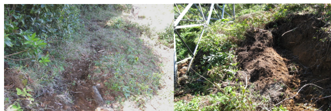
Fig.16. Fractures to the West of tower 62, obvious movement towards East, causing small landslides that put pressure on the structure. Picture from Geol. Ronald Valverde.
