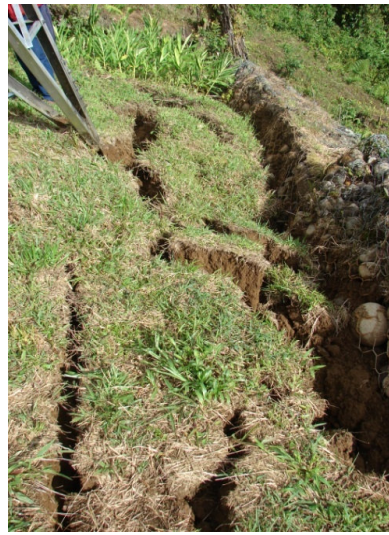
Fig. 7- Tower 37 LT Cariblanco – San Miguel. Horizontal and vertical movement in the terrain and structure. Picture from Ing. Bayardo Selva Mora.
