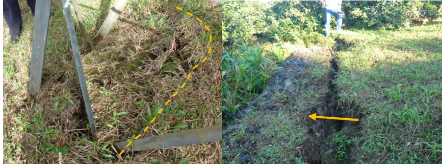
Fig.10. Tower 38 LT Cariblanco-San Miguel. Note the horizontal movement in the terrain and possible fracture. Ing. Bayardo Selva Mora. Y Cristiam Valerio
