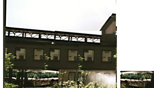
Figure 7-23: Two rectified photo images stored as one image file
